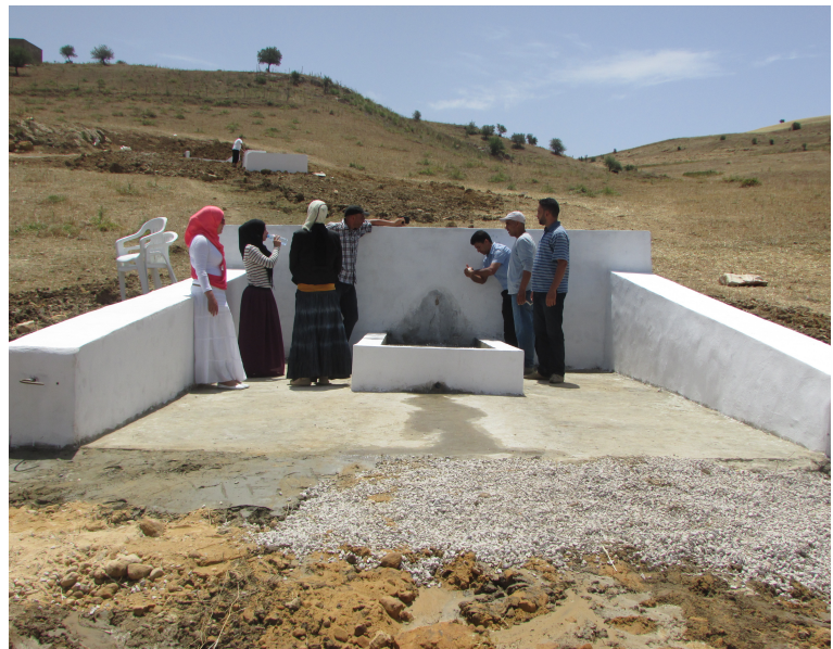
Nejb Ouerghi's completed water project.
